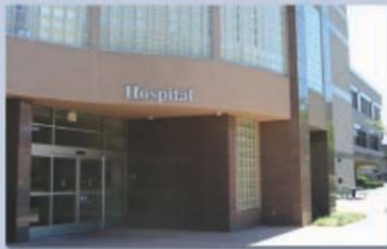
Wireless Sensors at Hospitals
